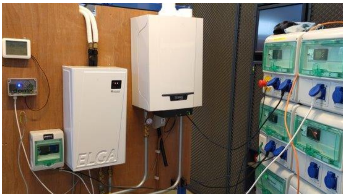
Figure 4: The hybrid heat pump setup in the HESI lab (Elga heat pump on the left and gas boiler on the right)
