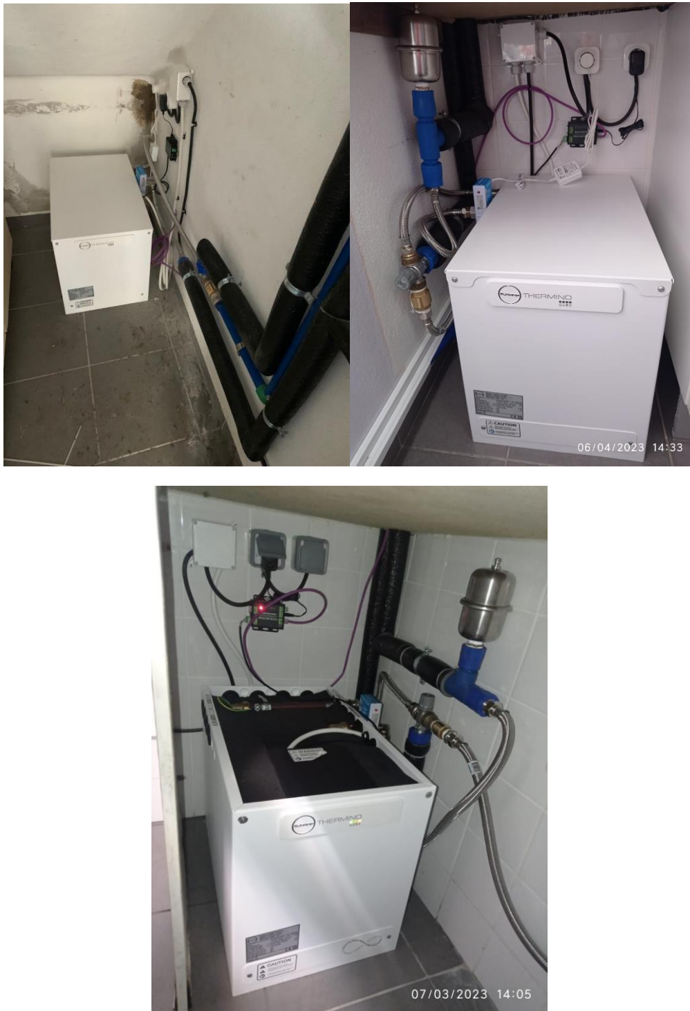
Figure 7: Heat-battery installations in Terceira.
