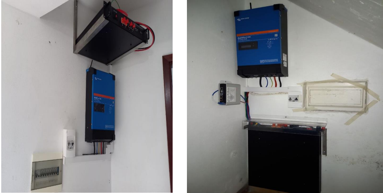
Figure 23: Installation and commissioning of the Victron inverter.
