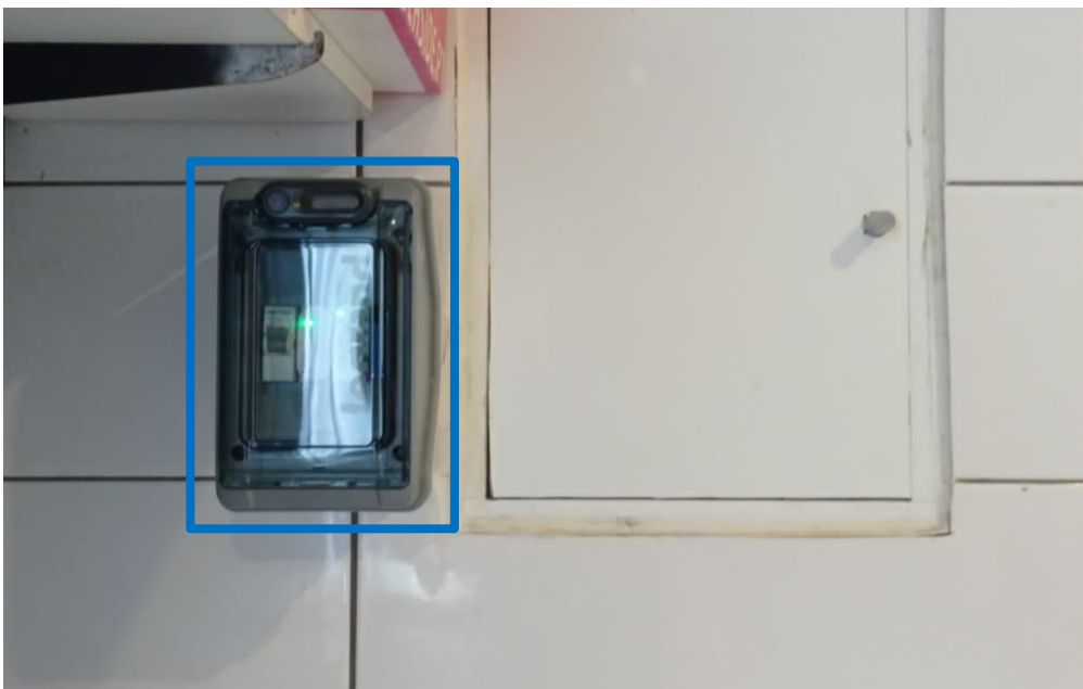
Figure 13: One of the installed switchboards for IANOS solutions' protective devices and meters (highlighted in blue).
